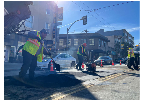
Pothole Repair
