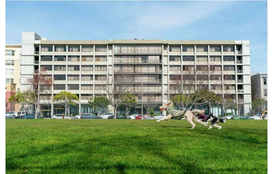
Source: SF Chronicle. This concrete building was recently retrofitted.
