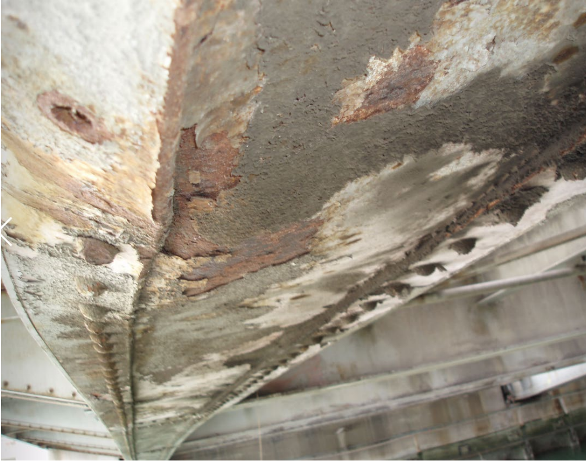
Deteriorated girders and deck – Structural deficiencies noted in Caltrans Bridge Inspection – Impetus for bridge rehabilitation in 2013
