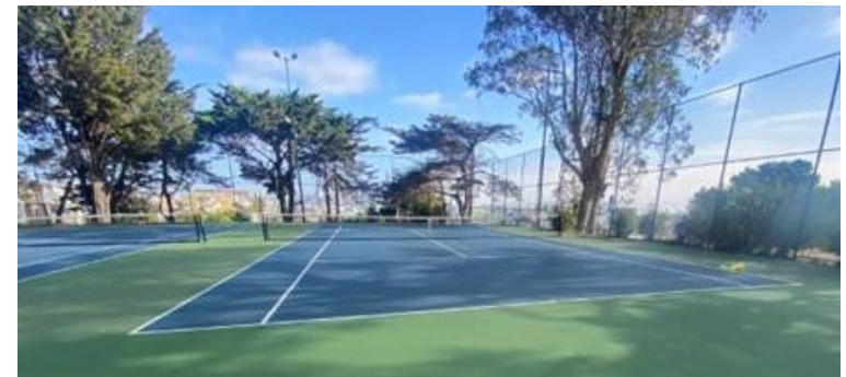
Potrero Tennis Courts Patching & Repainting
