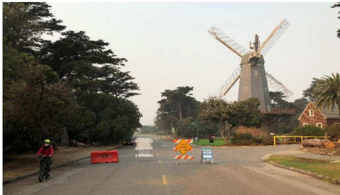
Park Roadways Repairs and Improvements
