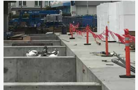
49 South Van Ness Construction
