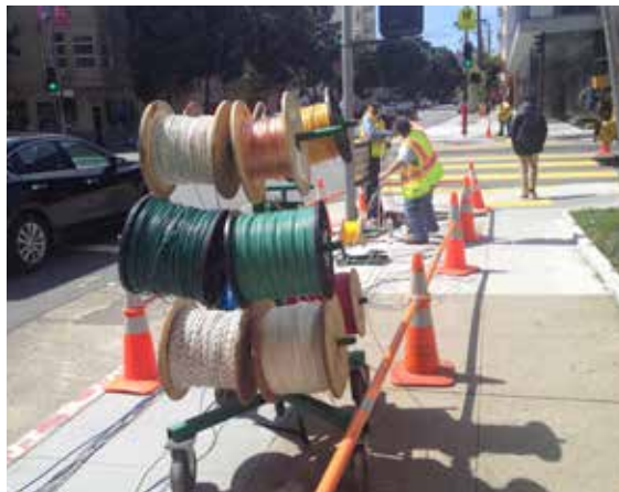
Fiber and WiFi Installation
