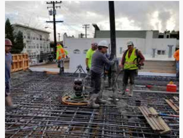
Fire Station Roof Replacement
