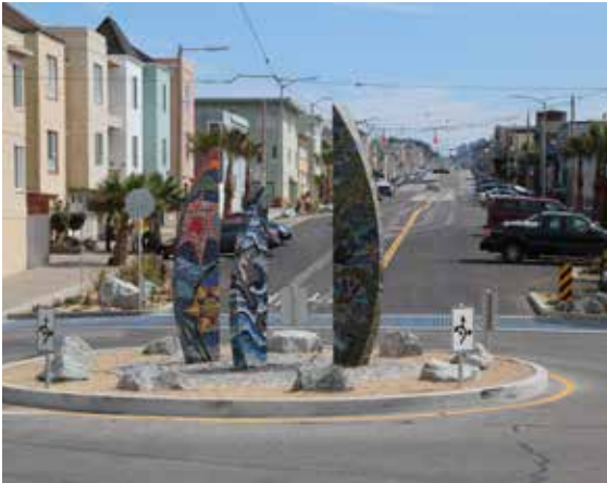
Recently Completed Taraval Streetscape Project
