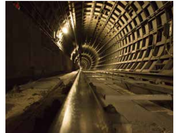
Muni Metro Tunnel
