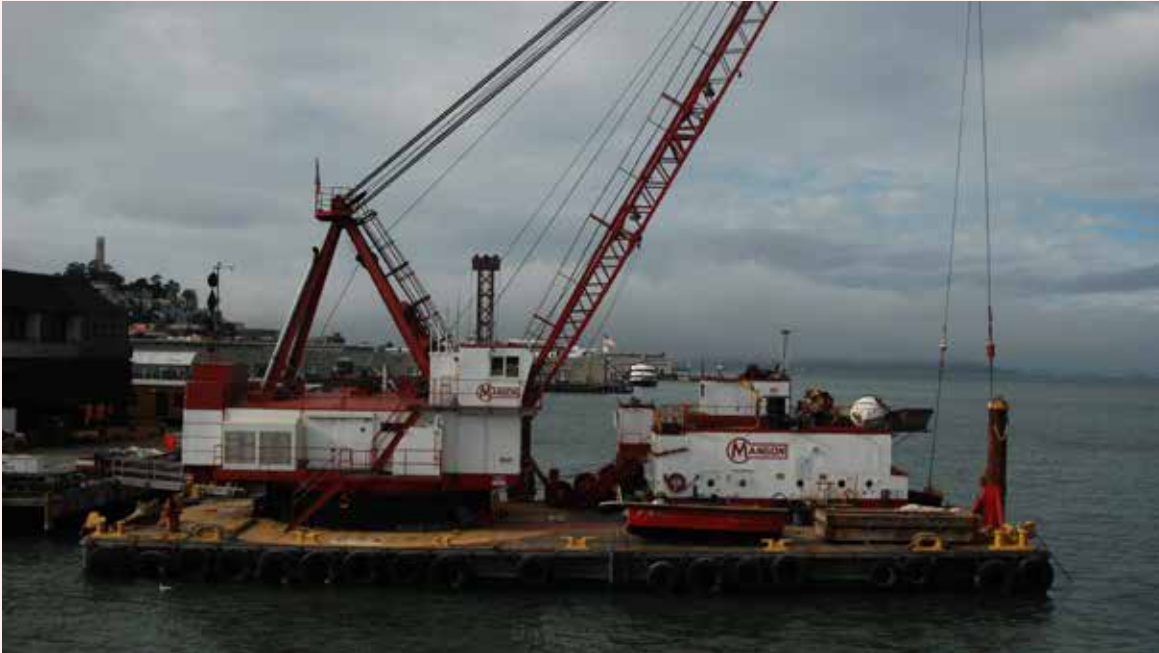
Dredging at the Port
