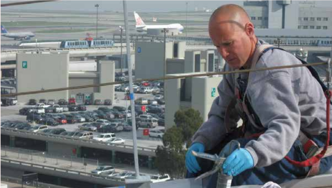
Roof Repair at SFO
