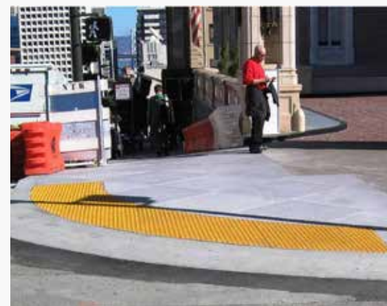
Newly Installed Curb Ramp
