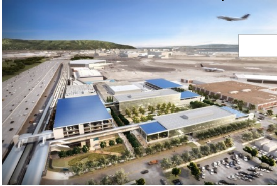
Consolidated Admin Campus
